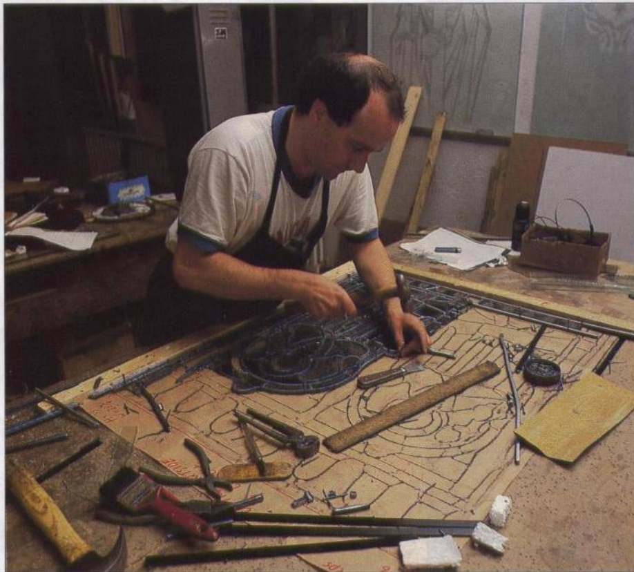
Peter McCrystal re-leading the 200-year-old window from St Mary's Cathedral, Limerick, using a crayon sketch.
